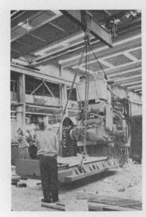
Numerically-Controlled Milling Machine is Installed
